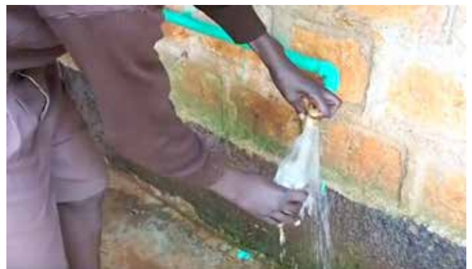
Preparation of clean drinking water
